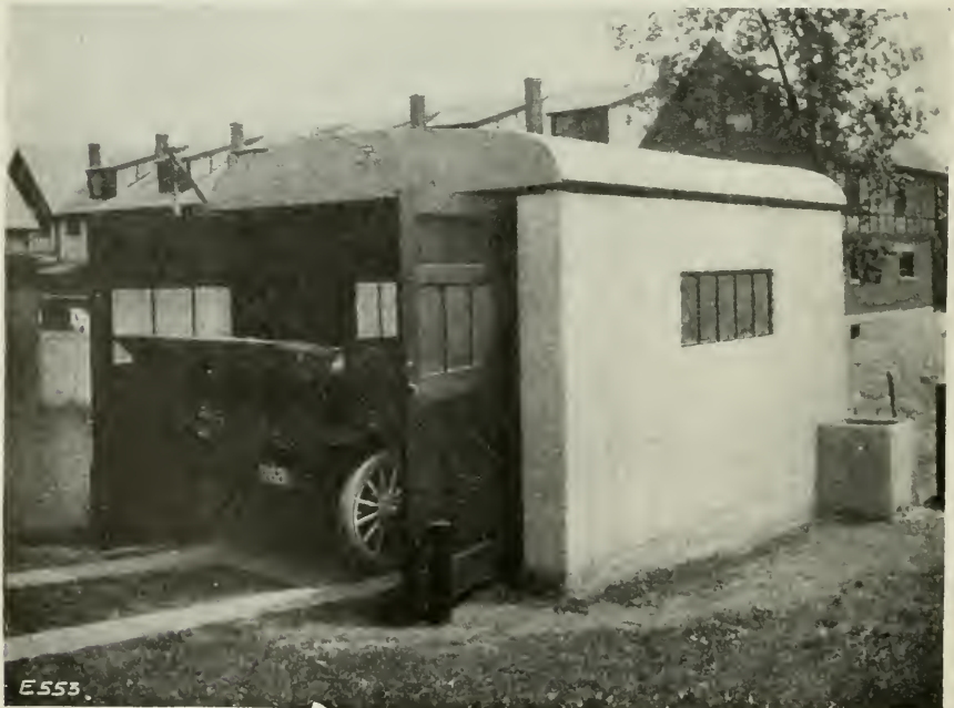
FIG. 54.—VIEW OF METAL LATH STRUCTURE COMPLETED.
